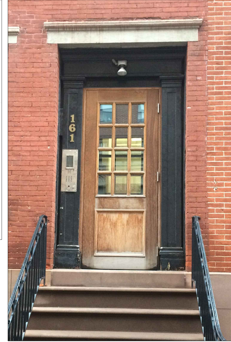
3 DOOR SURROUND AT 161 WEST 12TH ST. L-006
