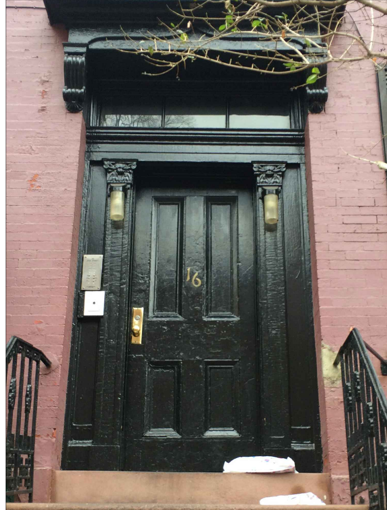
7 DOOR SURROUND AT 16 BANK STREET L-006
