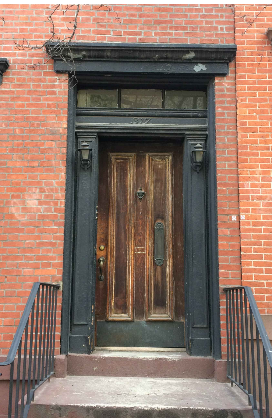
1 DOOR SURROUND AT 317 WEST 4TH ST L-006
